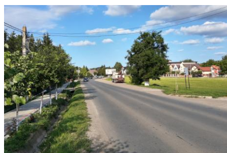
Fig. 4 – Constantin Langa Street with deleted road markings.
