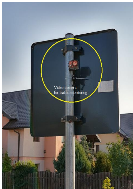
Fig. 9 – Video camera for traffic monitoring.
