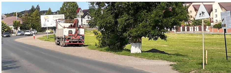
Fig. 5 – Street Constantin Langa with road markings erased.
